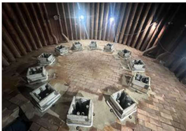
Figure 1: FREE JET Gen 3 burners installed in an operating unit.
